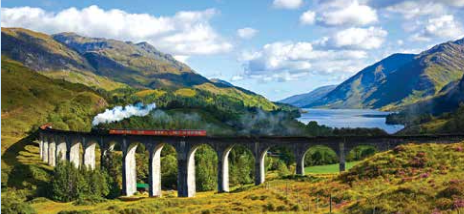
Winding through the austere Scottish Highlands, the 21-arch Glenfinnan Viaduct frames Loch Shiel, where steep slopes reflect into the loch's sparkling freshwater.
